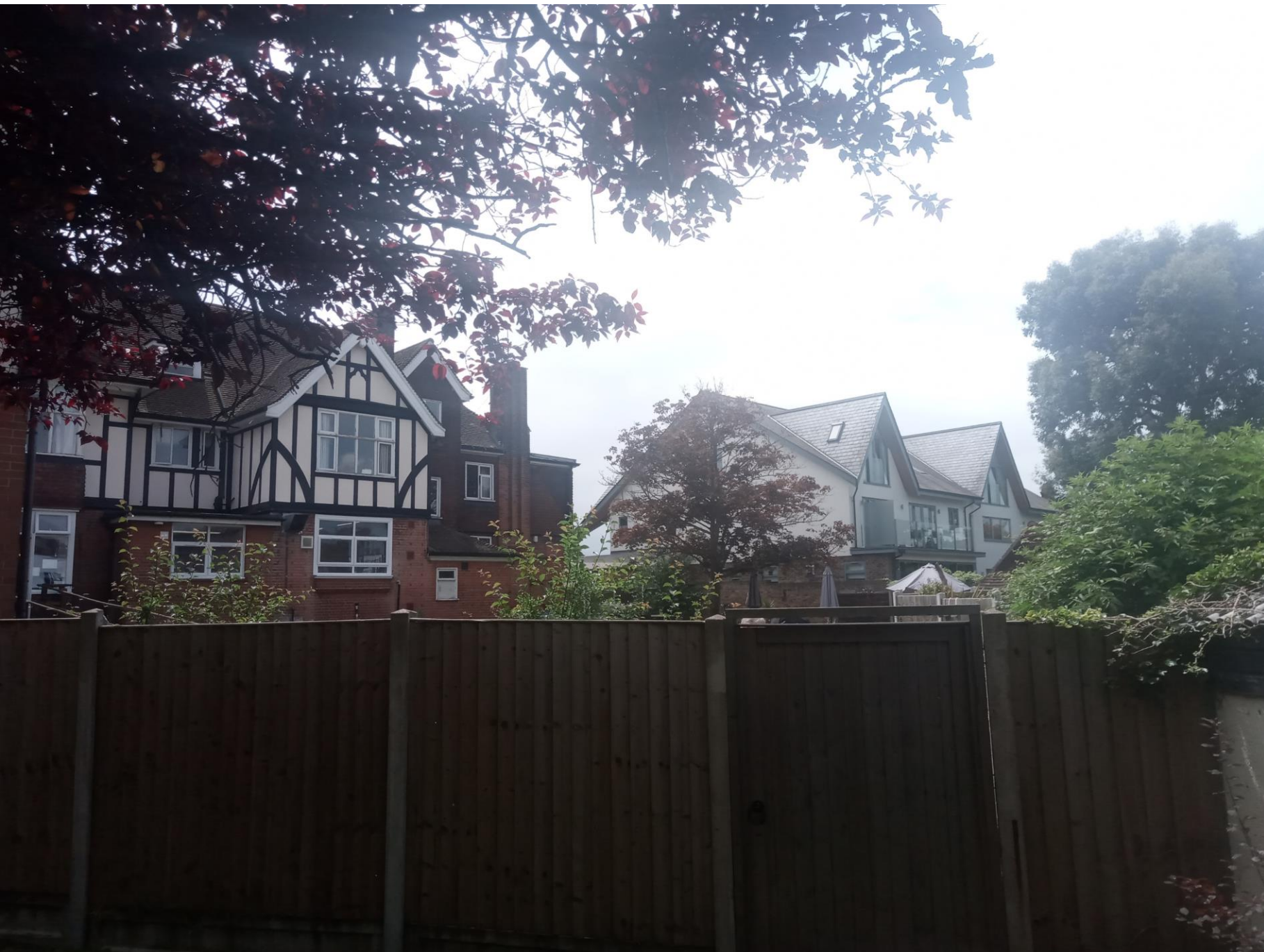
View to existing rear elevation of the application site
